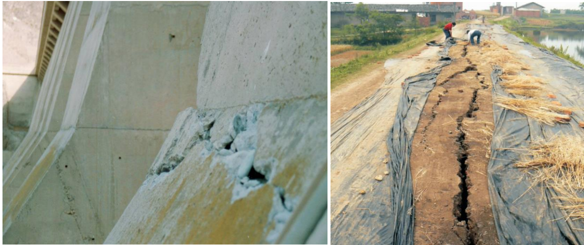
Figure 1: Crack in Sefid Rud buttress dam caused by the 1990 Manjil earthquake in Iran (left) and cracks in embankment dam covered by plastic sheets following the 2008 Wenchuan earthquake in China (right)
