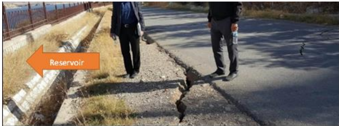
Figure 10 Sliding at the left abutment (adapted from directorate of Darbandikhan Dam).
