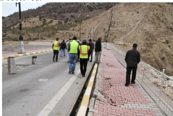
Figure 8 Longitudinal cracks and walkway deformation at the d/s side (looking to the left of the dam (Darbandikhan dam Directorate)).
