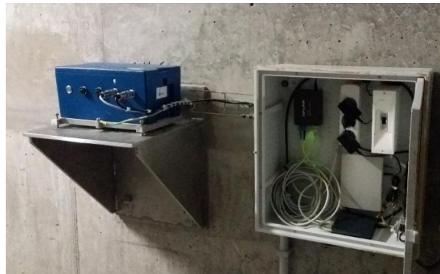
Figure 9: Seismic station in dam's galleries
